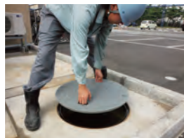
Reduction of risk by manhole weight reduction and reduction of working time
