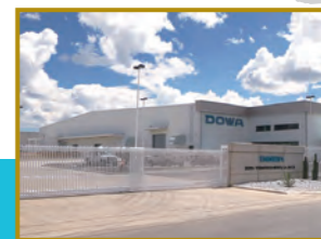
Heat treatment plant in Mexico
