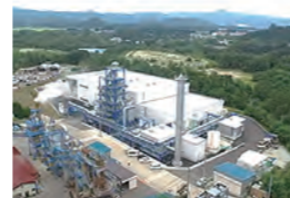
Low Concentration PCB Waste Detoxification Treatment Facility (Ecosystem Akita)
